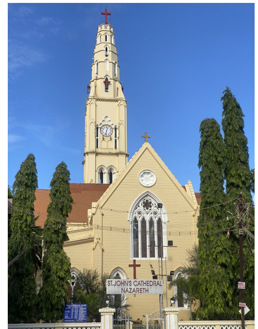
St. John's Cathedral, Nazareth, south end and transept.
